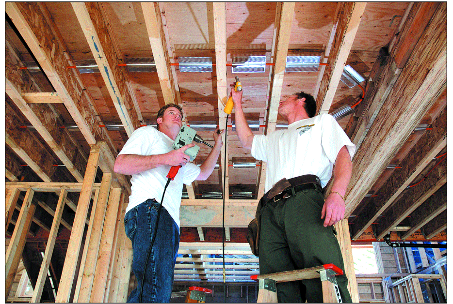
The Ultra-Fin radiant system requires fewer loops than a comparable staple-up system, saving time and money on installation. The system operates at 180°F and requires fewer manifolds and other hardware, yet can be zoned for greater comfort.
